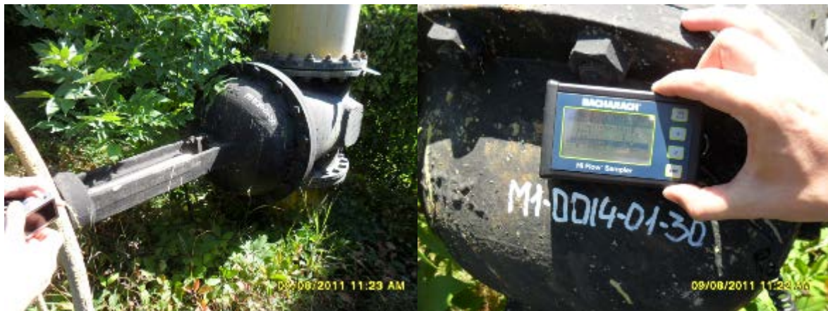
Figure 5 A Stand-Alone Valve with Stem Packing
