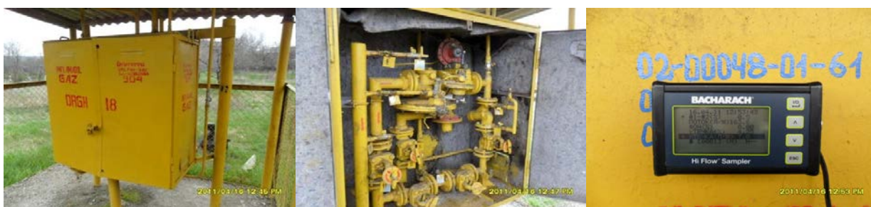
Figure 3 A cabinet type gas regulation point
